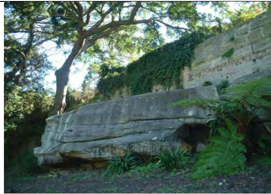
Figure S24 – Part of the sandstone block retaining wall resting on the rock bench which together support the grounds of the properties to the north of the Park. Photo: MWA, 2005.
