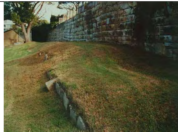
Figure S30 – Remains of sandstone foundations for former Park weatherboard changing sheds below the main block wall that supports the gardens of the properties fronting Louisa Road. Photo: MWA, 2005.
